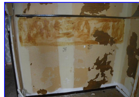
Joints de Placoplatre
